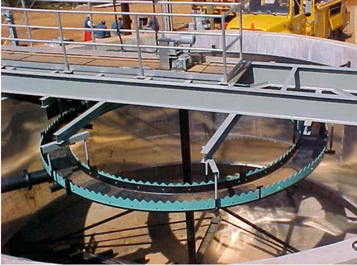
Typical bridge-supported peripheral feed clarifier.
