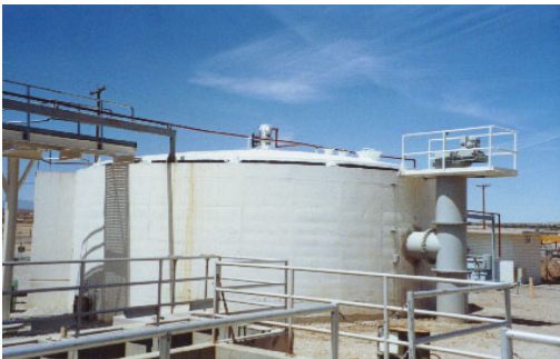
Typical radial beam fixed cover.
